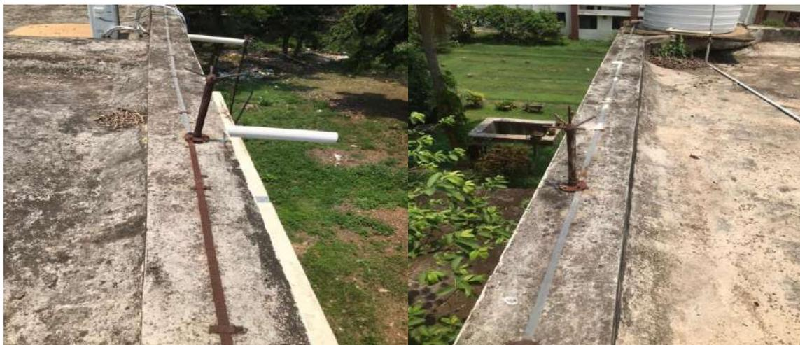
**Fig. 50 – Lightning Arrestors in the Terrace of Institute’s Main Building and D.M.School Building**
